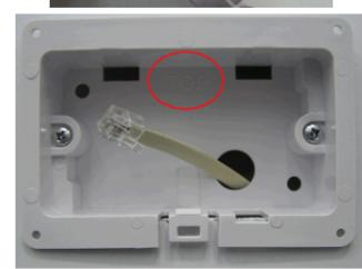
Feed the communications cable through the rear hole, fit the Screen Back into the wall (Note that the TOP marking should be at the top), then tighten the screws. Your mounting frame is now ready to accept the screen.
